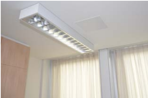
Figure 7: Opticlean installed in a gypsum board ceiling
